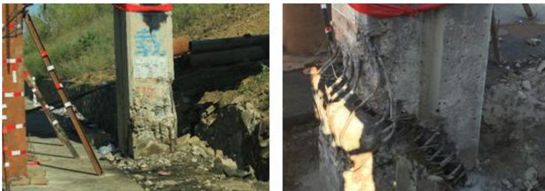
Fig. 2 - Damage characteristics of the pier of the G1011 Ha-Tong high-speed K302+095 separated overpass
