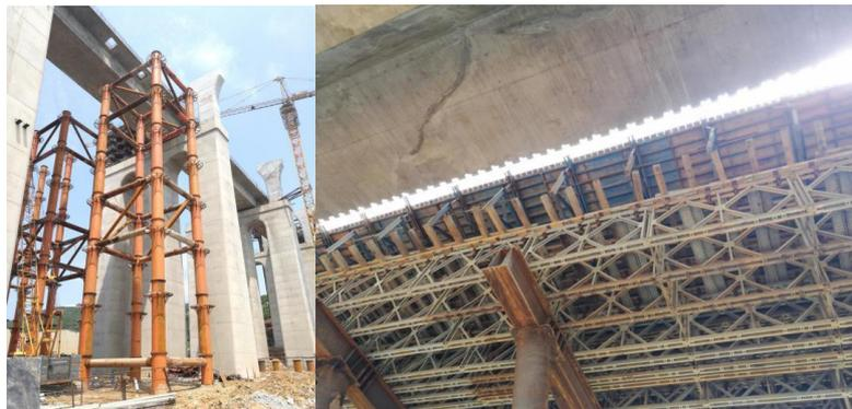
*Fig. 1 - On-site bracket support system*
