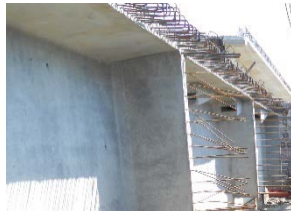
(c) Anchorage details on the field
