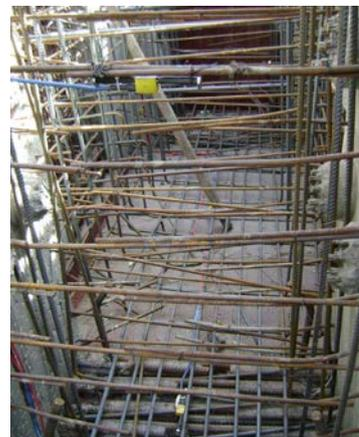
(b) Strain gage impeded in the connection
