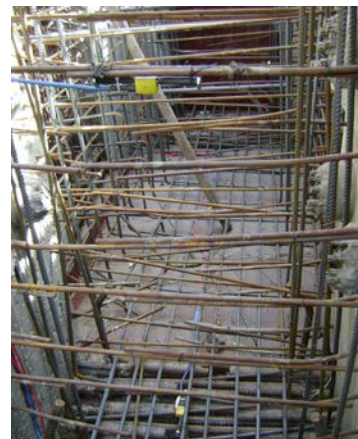
(b) Strain gage impeded in the connection
