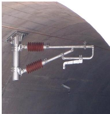
Fig. 3 - Bolt type contact net hanger after installation
