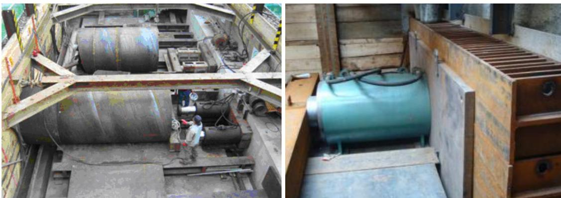
Fig.6 - Pipes jacking
