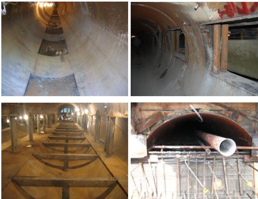
Fig.7 - Cutting, supporting and concrete pouring
