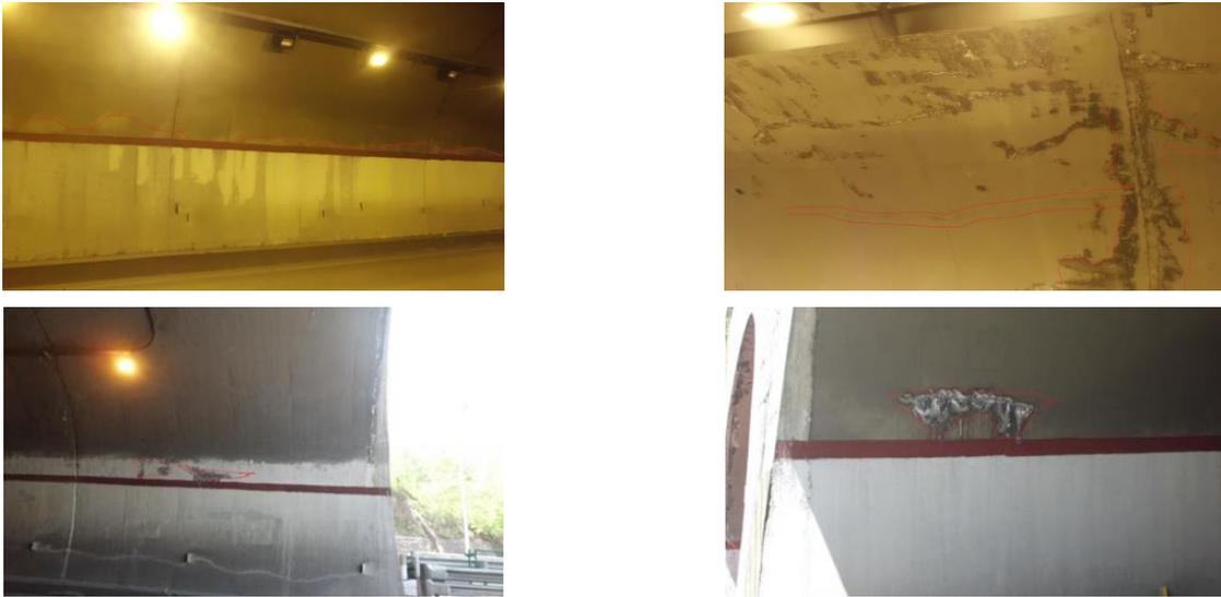
*Fig. 3 - Vertical linear water seepage*
