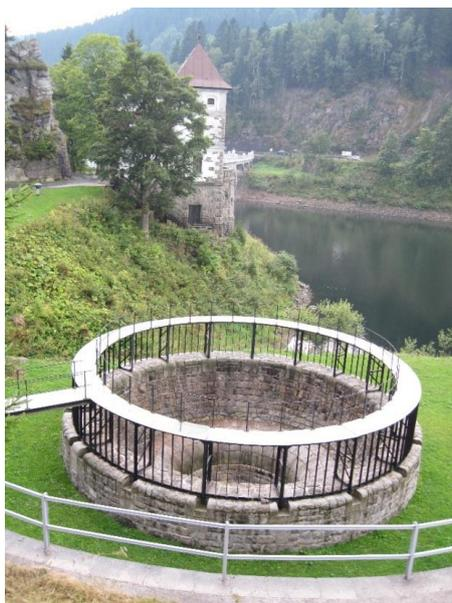
Fig. 1 - Shaft spillway in the Labská Dam
