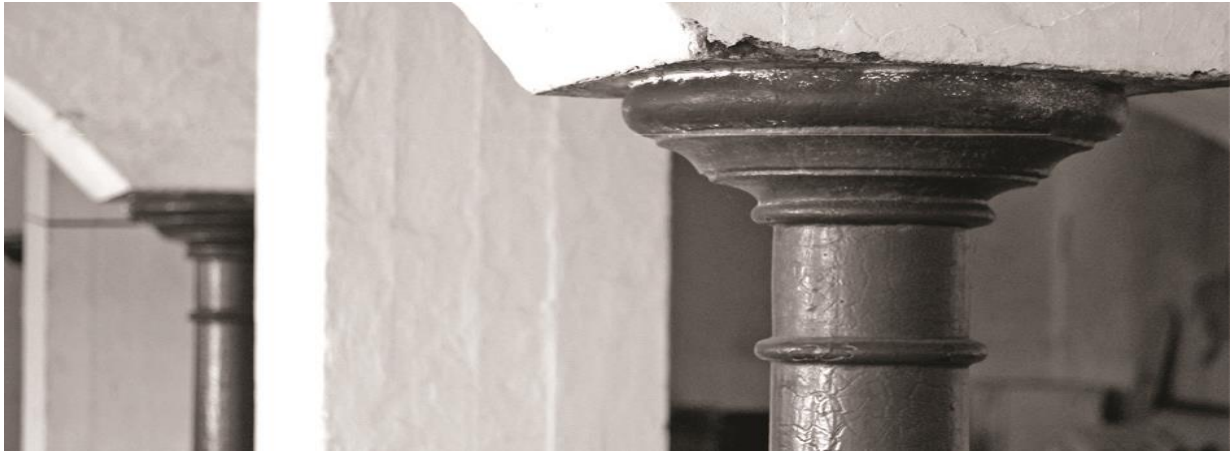
Fig. 4. Cast-iron columns in brewery building in Kralupy nad Vltavou (author's photo)
